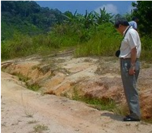
Plate A9-1 Surface Erosion
